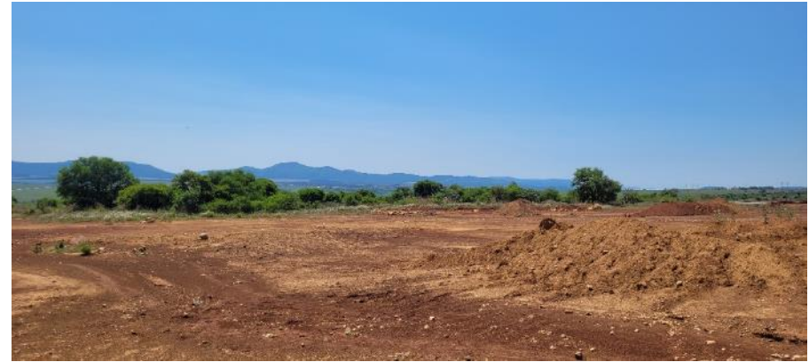
Large scar of cleared vegetation and exposed soil (bare land).
