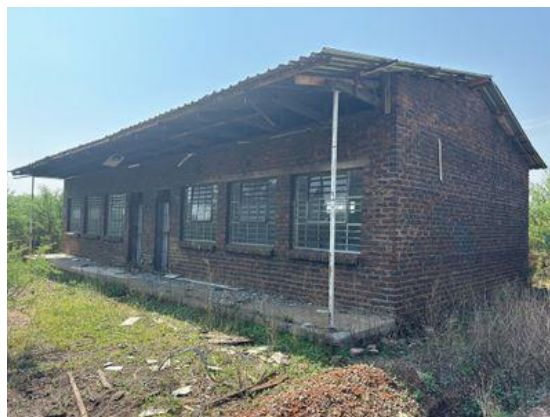
Figure 16: School building at LS003
