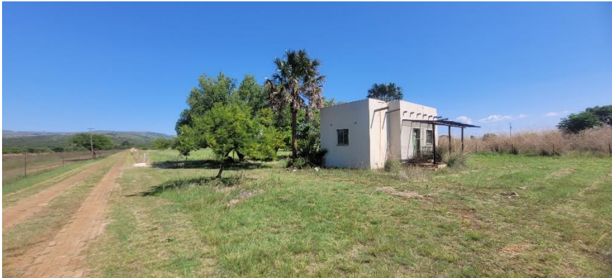
Existing building structures.
