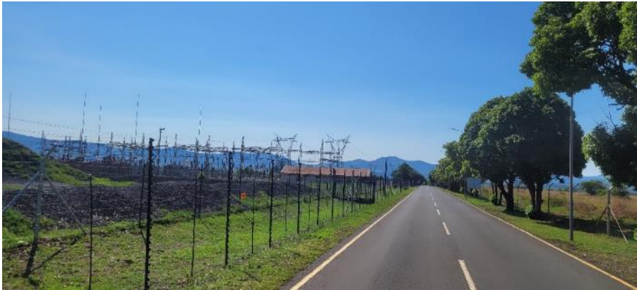
Main access road and existing services including Eskom Switching station.
