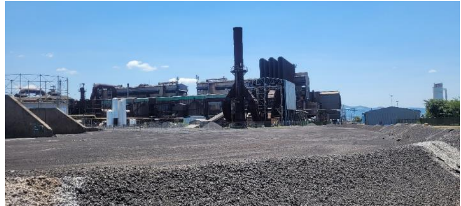
Smelter Plant, currently non-operational.
