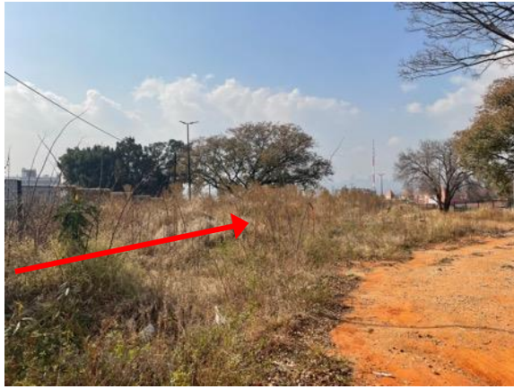
Figure 2 – Start of the pipeline as it runs east towards Jan Smuts Avenue
