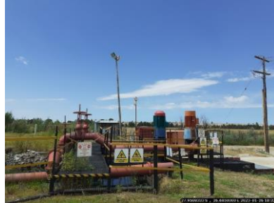
Existing pump station infrastructure
