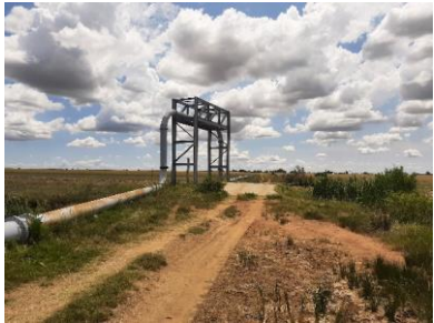
Existing pipeline road crossing
