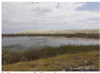
Tailings storage facility and return water dam
