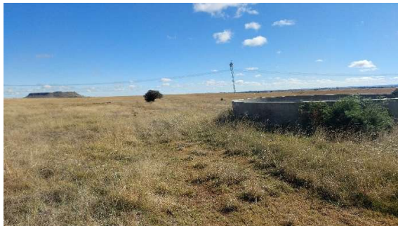
Figure 5: Multiple concrete dams found on-site.
