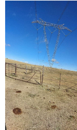
Figure 6: Powerlines crossing ER 94.
