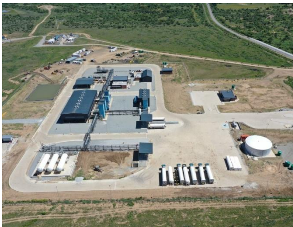
Figure 17: Helium / LNG Plant construction area as of 22 nd February 2024.
