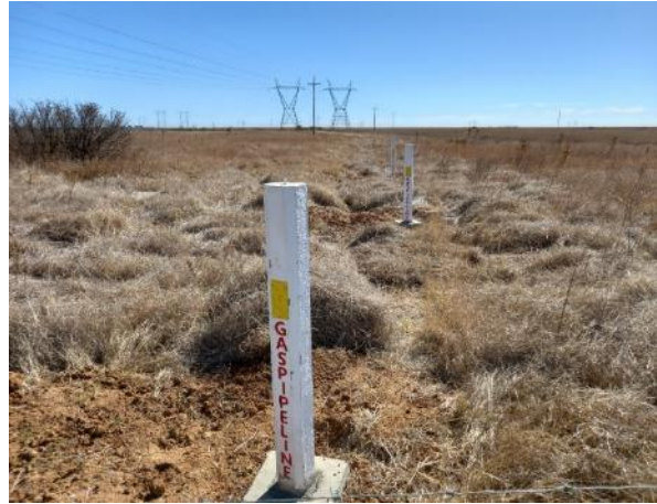
Figure 14: Rehabilitated pipeline route.
