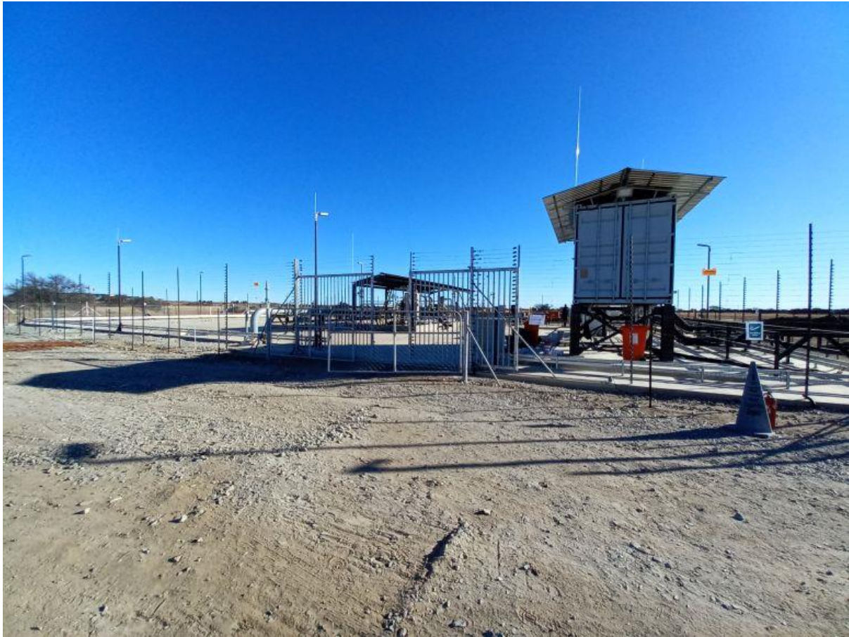
Figure 6: View of existing in-field compressor site.
