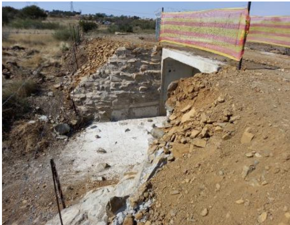
Figure 15: Culvert on access road.
