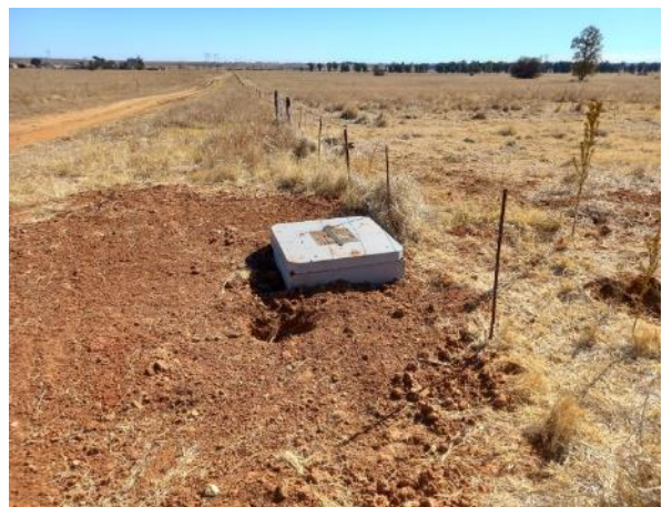
Figure 12: Low point drain.
