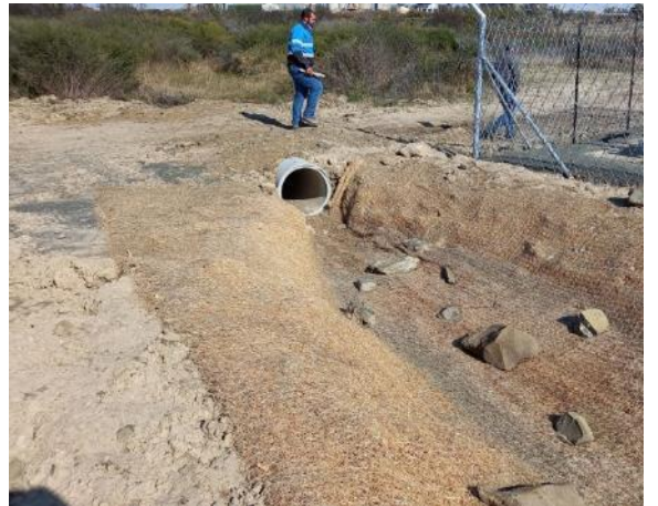
Figure 16: Flume pipe on access road.
