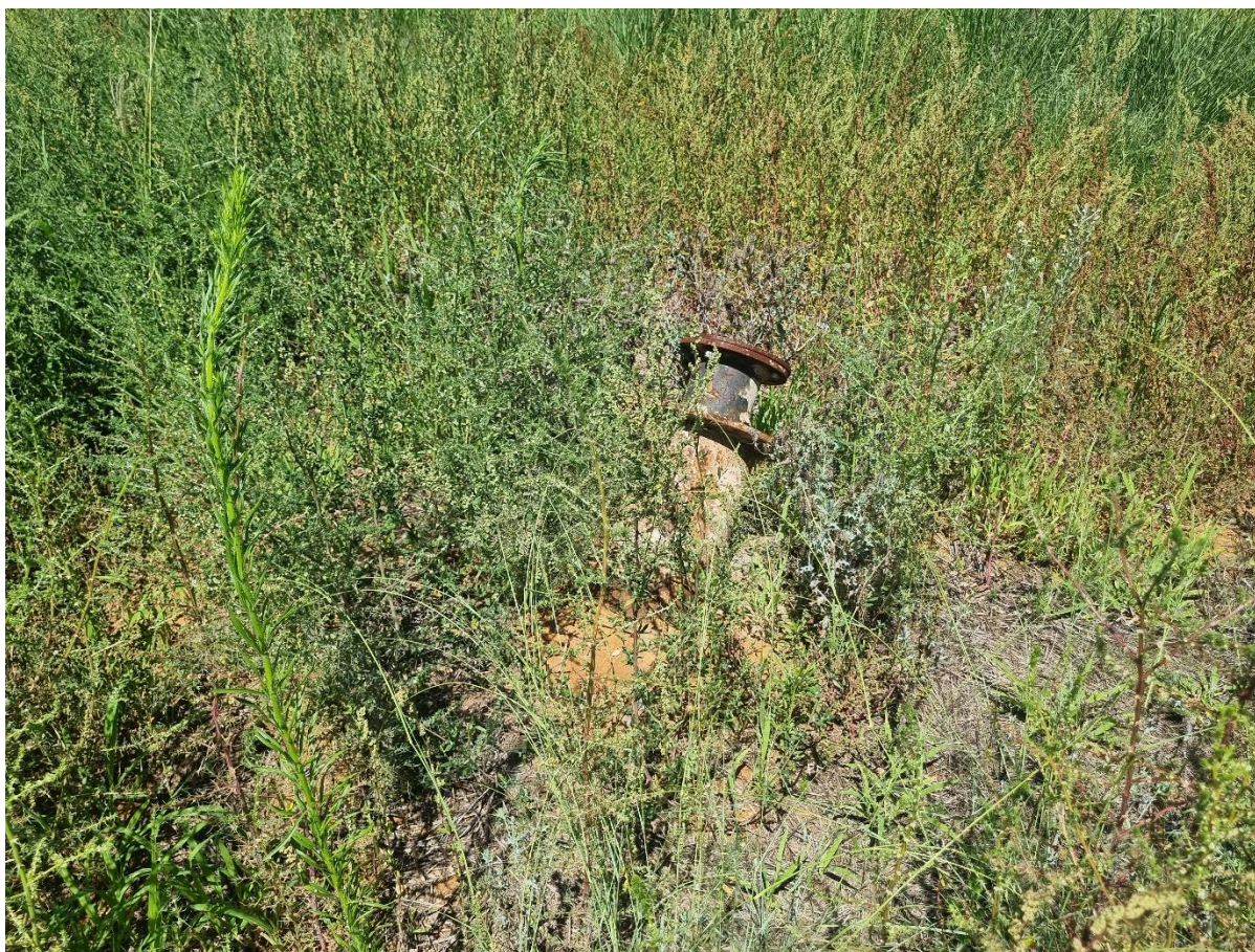
Figure 2: Example of a wellhead in the process of decommissioning, prior to being cut.
